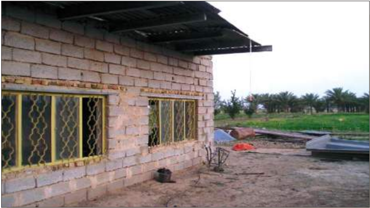
Figure 2 — Example of Typical Baghdad Construction
